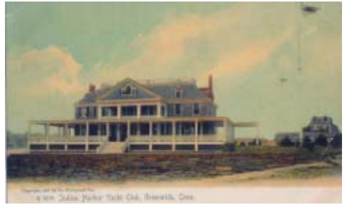
The Indian Harbor Yacht Club From the end of the Pier
